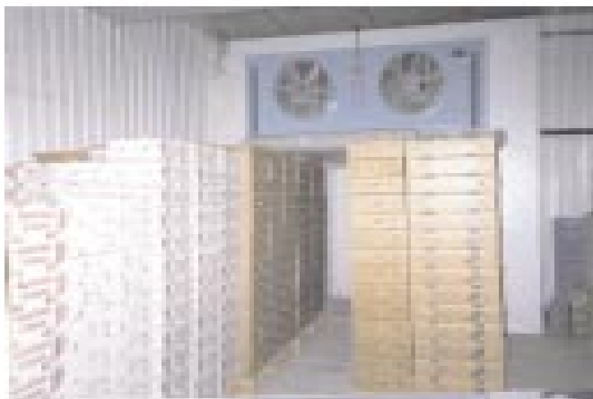
Photo 2: Tunnel arrangement showing cooling coil, packed grapes ready for precooling and tarp rolled up.
