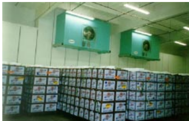
Photo 3: After precooling grapes are stored in a cold storage maintained at 0^{\circ}\text{C} & 90% RH ready for loading in refrigerated container for the journey by road to Mumbai port.
